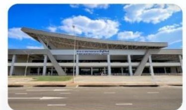
Underground (Buriram, Roi Et Airport)
